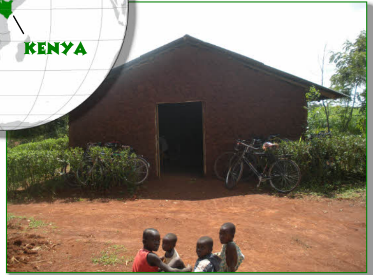
Above: Ganga Village, Kenya. The church building that was built with a DMI donation in 2001.
